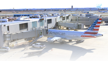
Philadelphia International Airport Passenger Boarding Bridges
