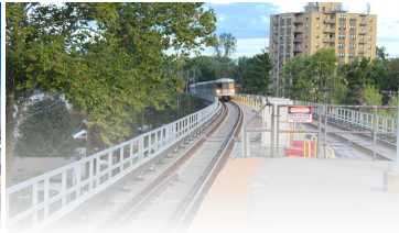
DRPA PATCO Westmont Viaduct
